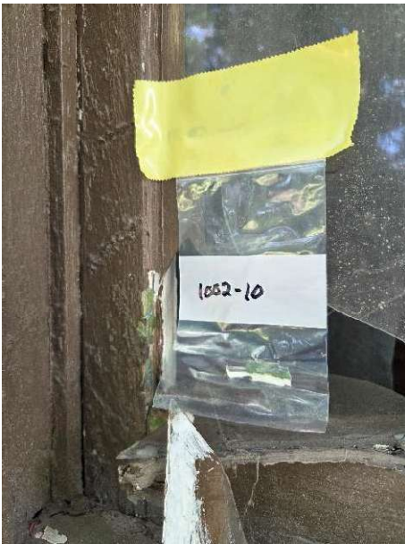
Sample 1002-10 Typical Exterior Caulking Sample
