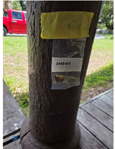
Sample 1002-07 Typical Stucco Sample
