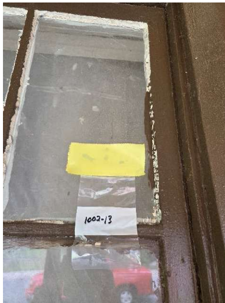
Sample 1002-13 Typical Window Glazing Sample
