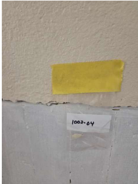
Sample 1002-04 Typical Wall Texture Sample
